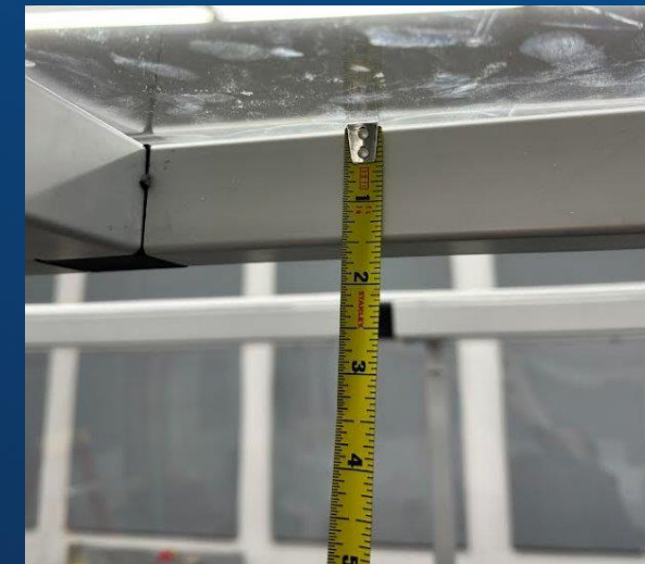
Figure 30: Deflection Point Testing
