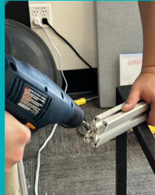
Figure 27: Drilling Holes into Truss
