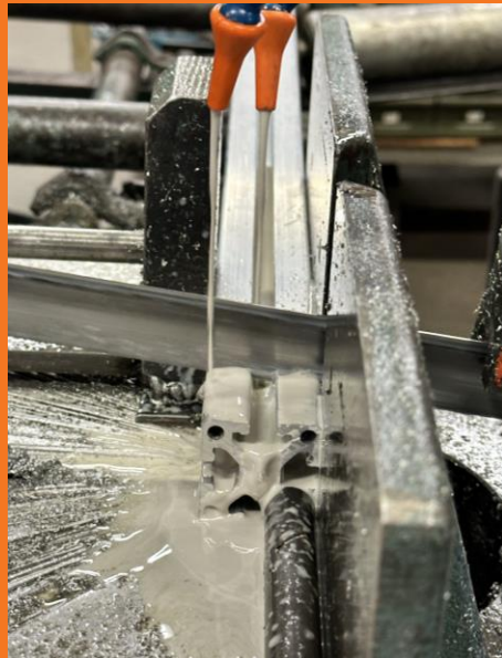
Figure 26: Support Beam Trimming
